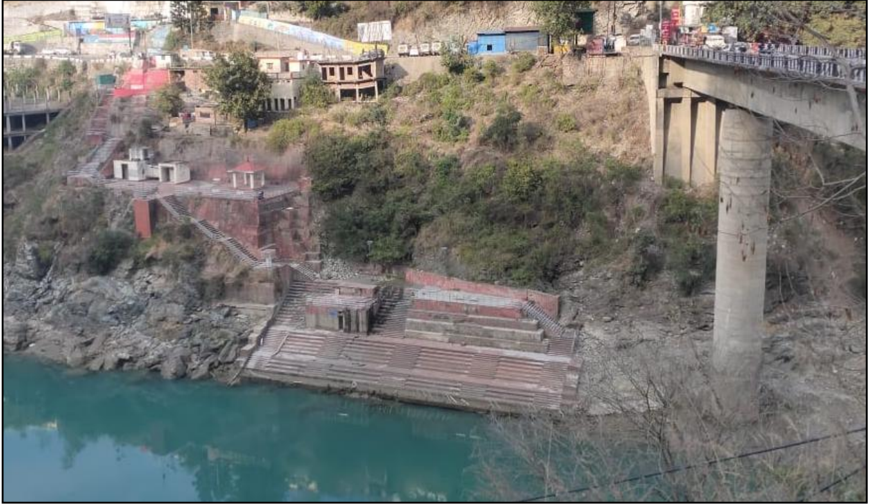
Figure 5.11: Damaged and neglected ghat near Kirtinagar
