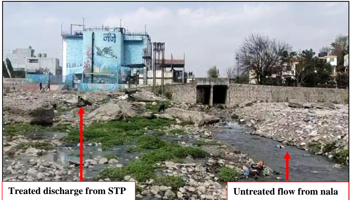
Figure 5.6: Part flow of nala treated by STP while balance remains untreated. Both joining the Ganga at Muni-ki-Reti, Rishikesh
