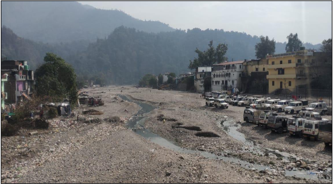
Figure 5.7: Construction in floodplain and nala bed in Rishikesh (Picture by author)
