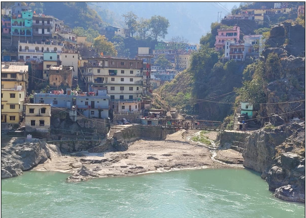
Figure 5.8: Houses on immediate riverbank at Rudrapryag (Picture by author)
