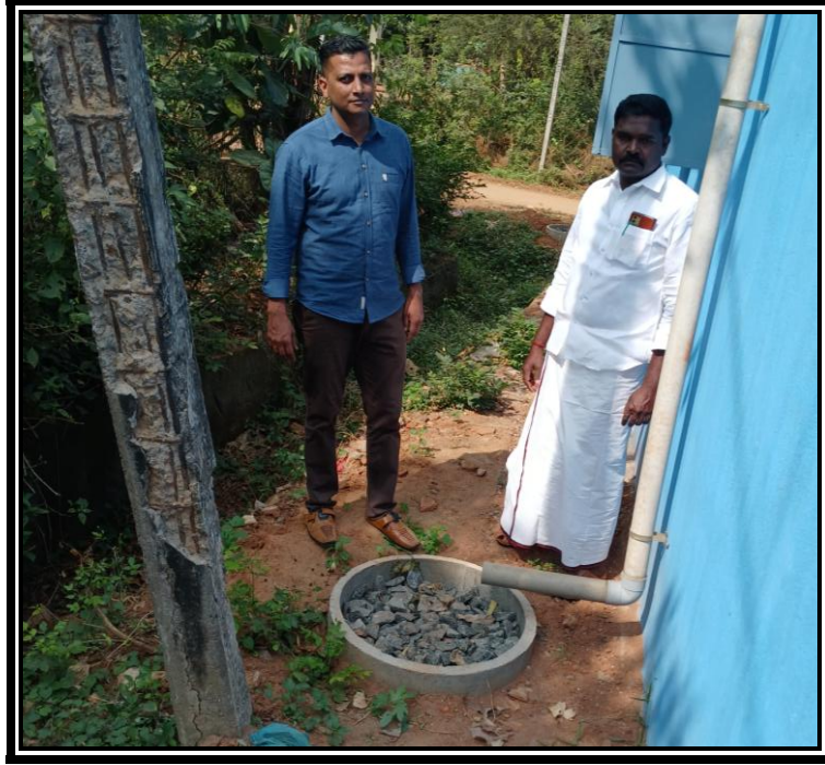
Soak Pit constructed in Aganwadi at Mattangal Vilage of Pudukkottai District
