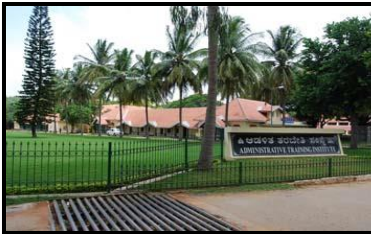
Figure 41 Mysuru ATI (Source: ATI Mysuru Official Website)
