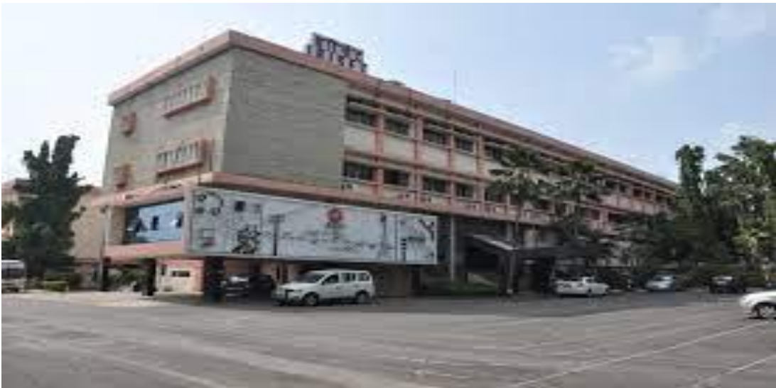
Fig 6. Indian Railway Institute of Signal Engineering and Telecommunication, Secunderabad
