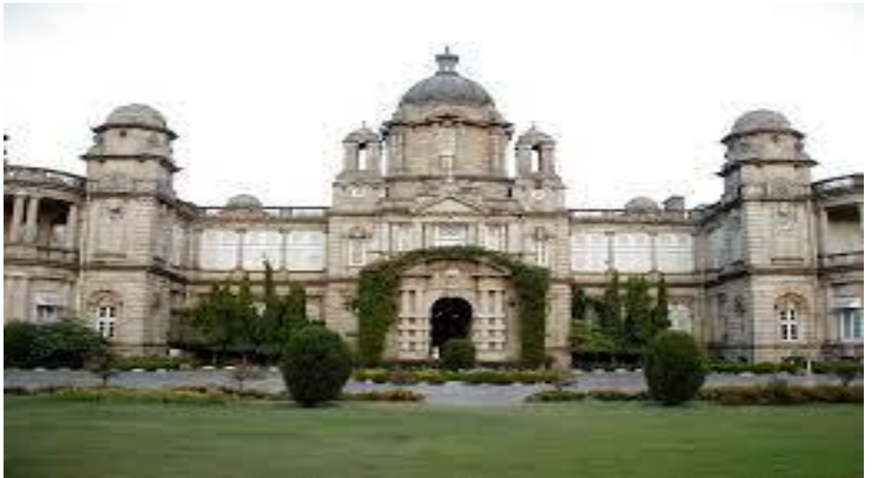
Fig 1. National Academy of Indian Railways, Vadodara, Gujarat
