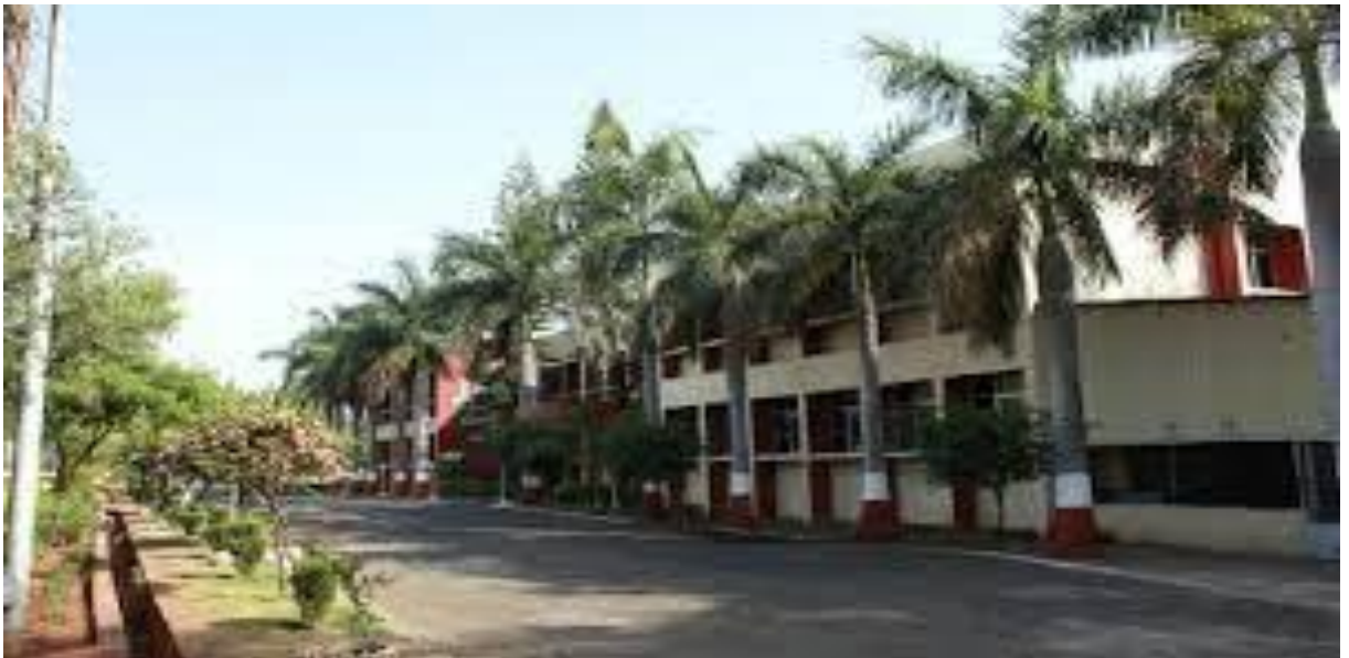
Fig 5. Indian Railway Institute for Electrical Engineering(IRIEEN)
