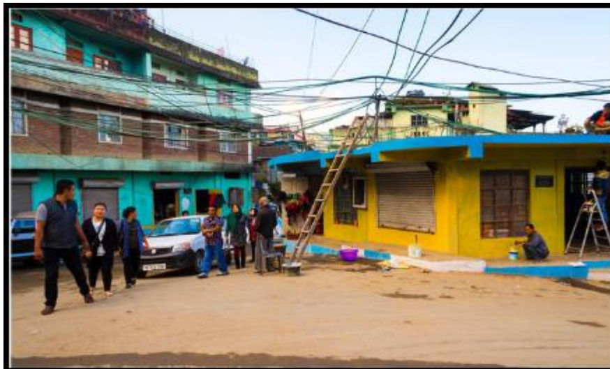
Fig 6-7: Lack of Space and Overburdened Electrification in Kohima (Dec 2022)
