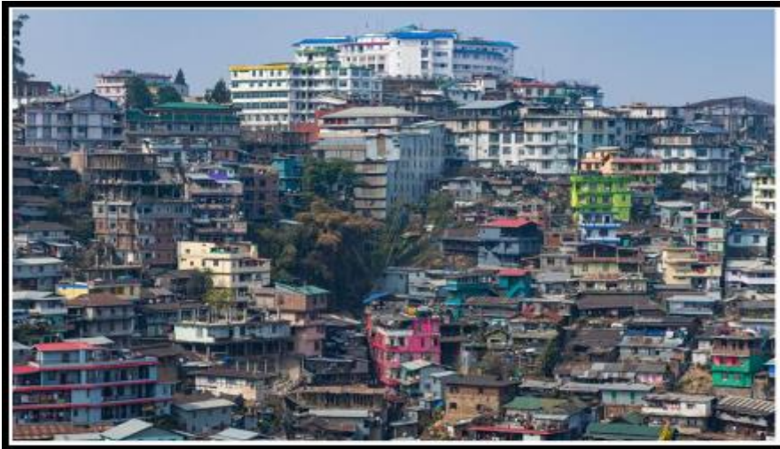
Fig 6-5: Lack of Space for Sewage and Sanitation in Kohima (Dec 2022)
