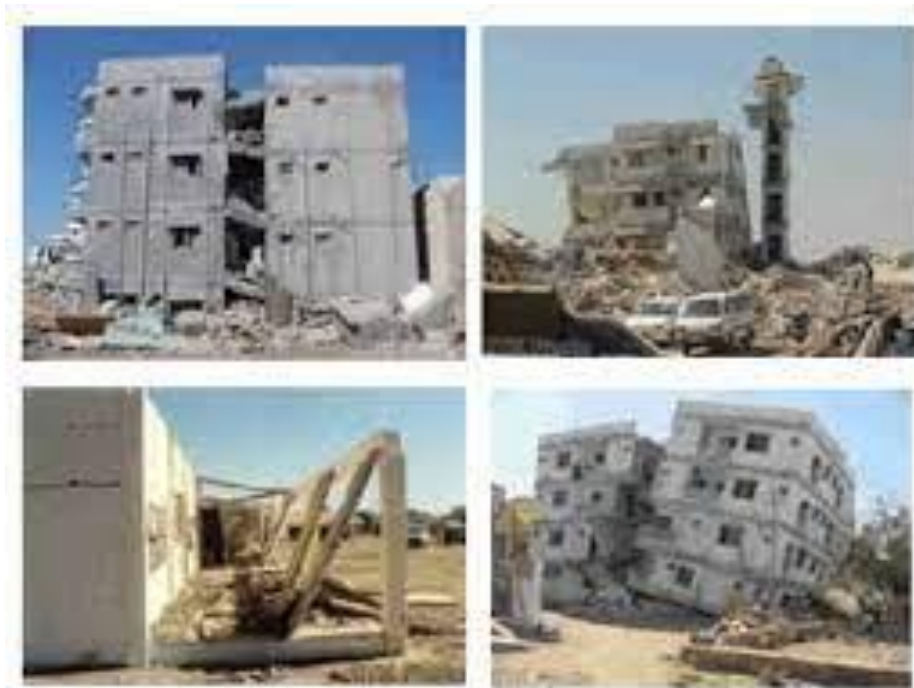
Fig 16 Some damaged Buildings in Earthquake
