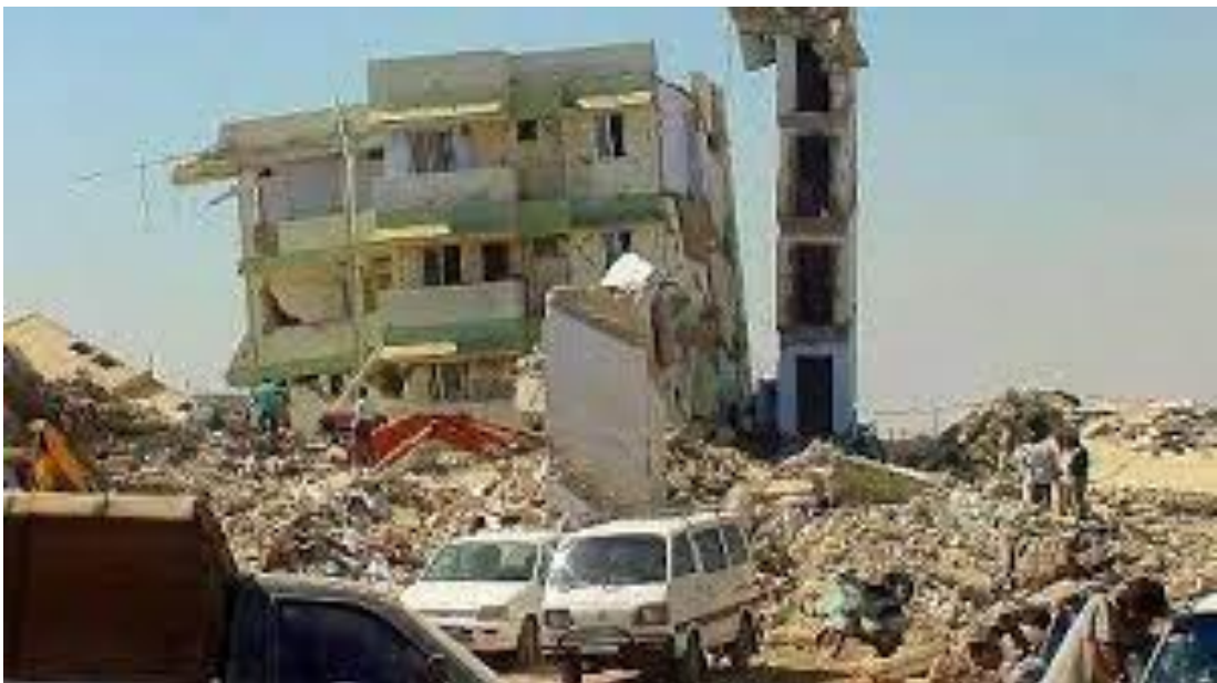
Fig 15 Damage in Earthquake
