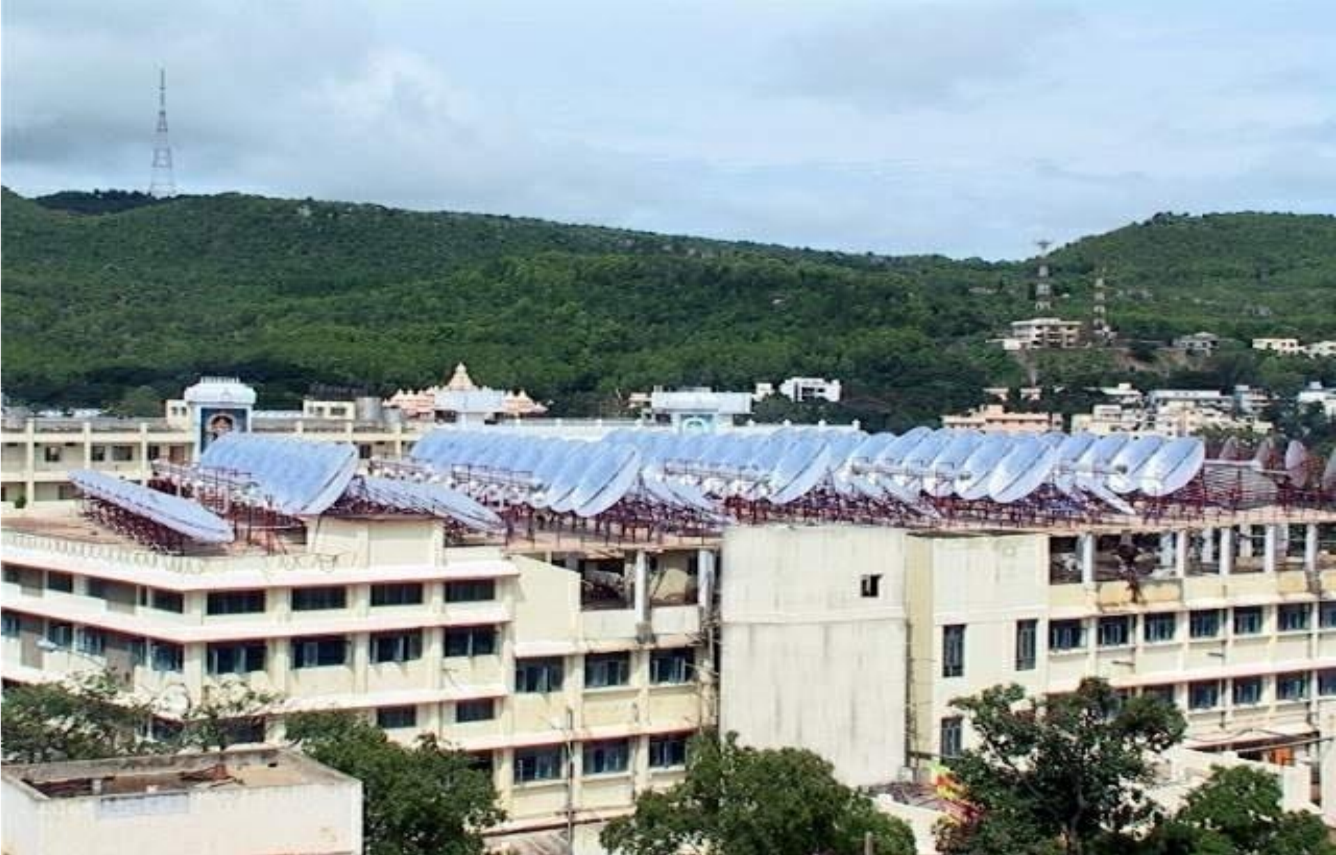
World's largest solar steam cooking system at a temple town of Tirupati for 15000 people
