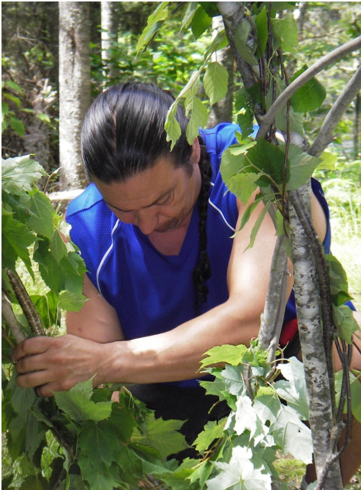
Fig. 1. Roger Paul ( Passamaquoddy ), bending saplings to construct the frame for a traditional Wampanoag wetu (dome-shaped shelter) beside the Penobscot River in Maine, during a Wabanaki Writers retreat in 2009.
