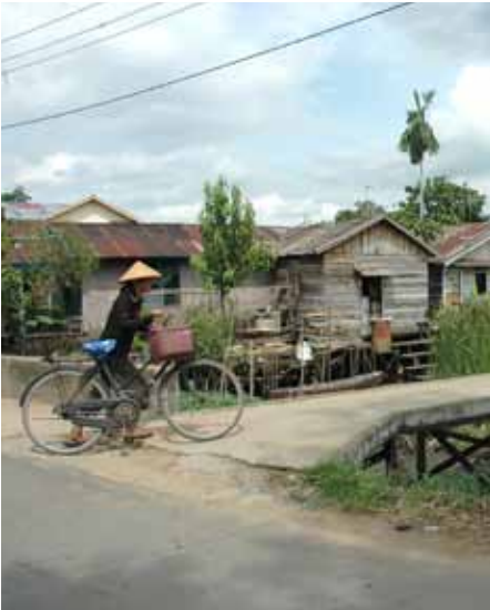
Footpaths provide safe access. Source: Ministry of Public Works.
