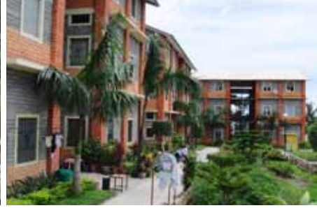
These apartments were built with community participation. Source: F. Steinberg.
