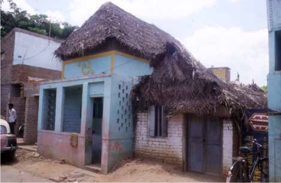
The "urbanism of hope," sites-and-services project, Chennai, Arumbhakam Source: F. Steinberg.
