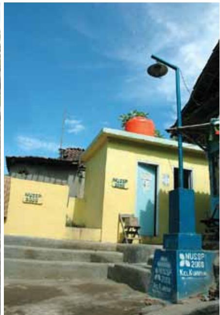
NUSSP community toilets, showers, and washing facilities Source: Ministry of Public Works.
