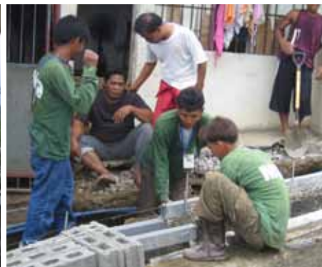
The STEP-UP project in Marikina: Building drainage infrastructure Source: F. Steinberg.
