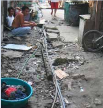
Preparing to replace informal water pipes Source: F. Steinberg.
