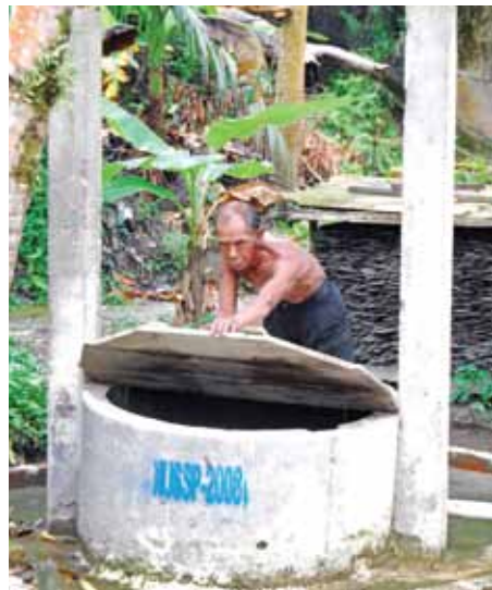
In more rural settings, water supply is still reliant on deep wells. Source: Ministry of Public Works.
