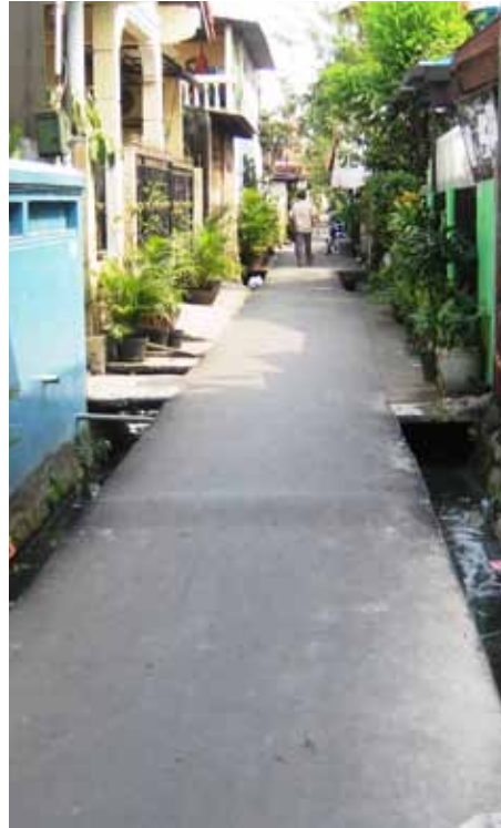
Jakarta, Gandaria Utara, Kebayoran Baru: Foot paths constructed as part of kampung improvement Source: L. Marulanda.
