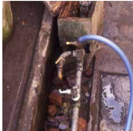
Jakarta: Kampung improvement included water connections to individual houses. Source: F. Steinberg.
