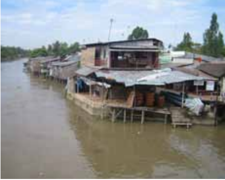
Can Tho: Informal housing along the Hau River Source: E. Kessler.
