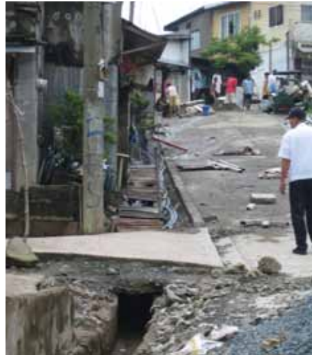
Marikina, Manila: Construction of alleys and drainage Source: F. Steinberg.
