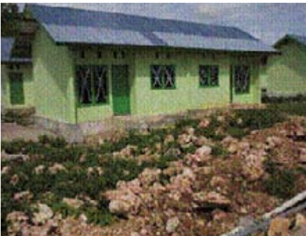
Bau-Bau, Sulawesi: Housing construction Source: Ministry of Public Works.
