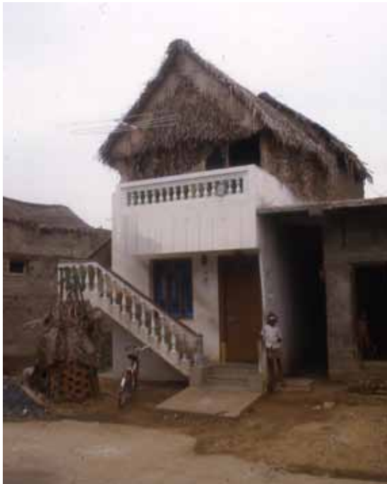
Consolidated homes in a sites-and-services project, Chennai, Arumbhakam Source: F. Steinberg.
