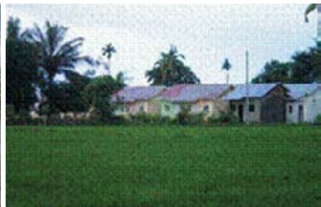
Watampone, Sulawesi: New site development Source: Ministry of Public Works.
