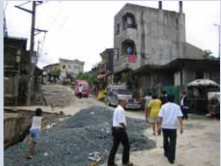
Improving road infrastructure Source: F. Steinberg.
