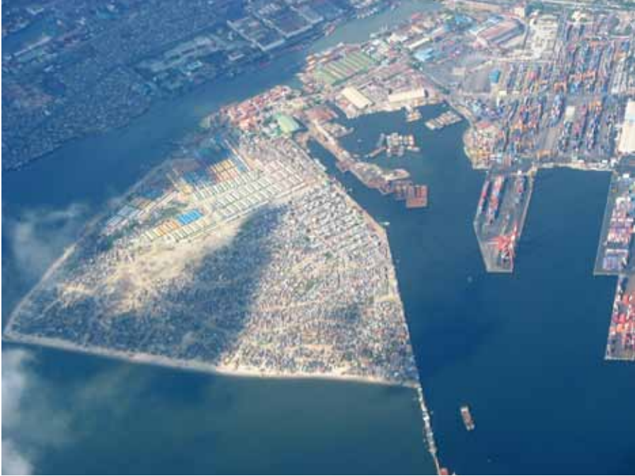
Baseco, Manila: A harborside land reclamation site that has become home to many victims of fires in Manila's informal settlements. New development, including massive informal settlements, has taken place despite the low load-bearing capacity of the site.
