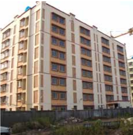
Mumbai, Maharashtra: Social housing Source: Ministry of Housing and Urban Poverty Alleviation.
