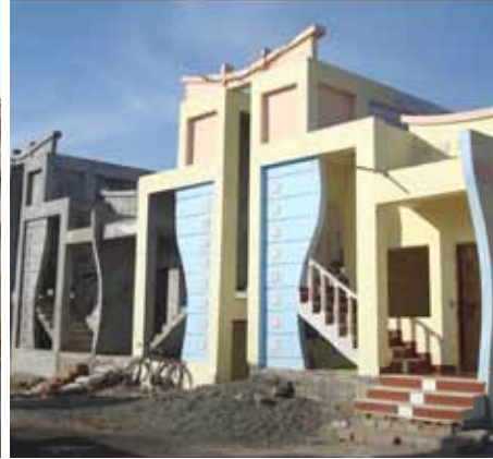
Indore, Madhya Pradesh: Social housing Source: Ministry of Housing and Urban Poverty Alleviation.
