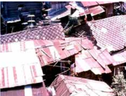
Bangkok: Baan Manangkhasila before land sharing and upgrading Source: CODI.
