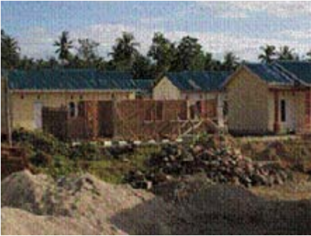
Polewali Mandar, Sulawesi: Housing construction Source: Ministry of Public Works.
