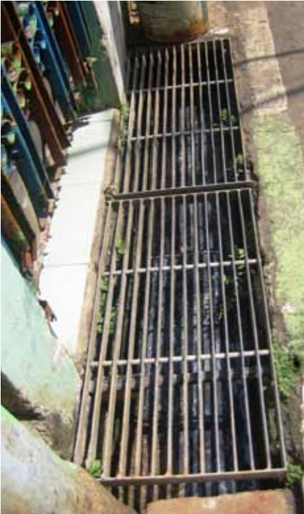
Jakarta, Gandaria Utara, Kebayoran Baru: Kampung improvement included construction of drainage works Source: L. Marulanda.
