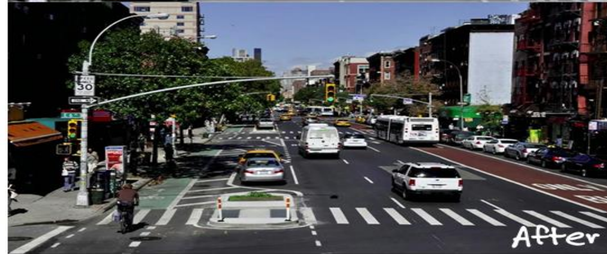
First Avenue Improvements, New York City
