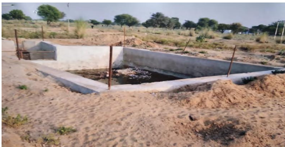
Photo : Recharge Structure Under Construction
