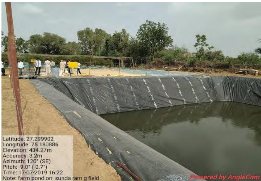
Photo: Farm Pond with Polythene Sheets to Prevent Loss
