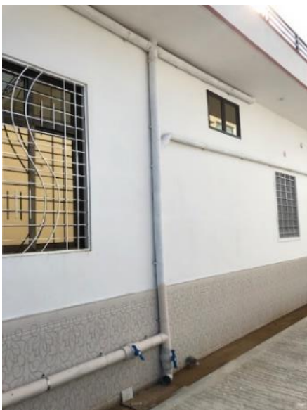
Photo: Rooftop Rainwater Harvesting System and Storage
