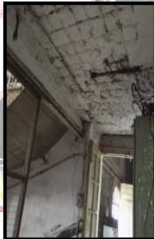
Deteriorated Roof Structure,GPO,Mumbai
