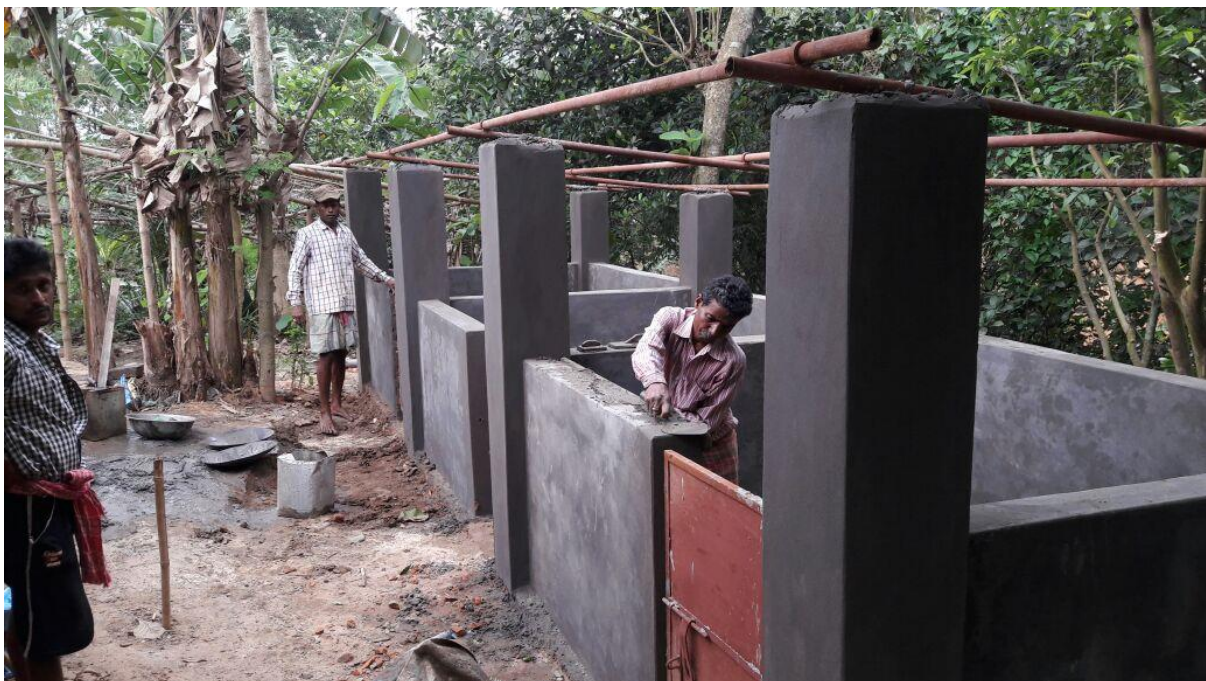
Figure 4.2 Pig shelter under construction in a JFMC
