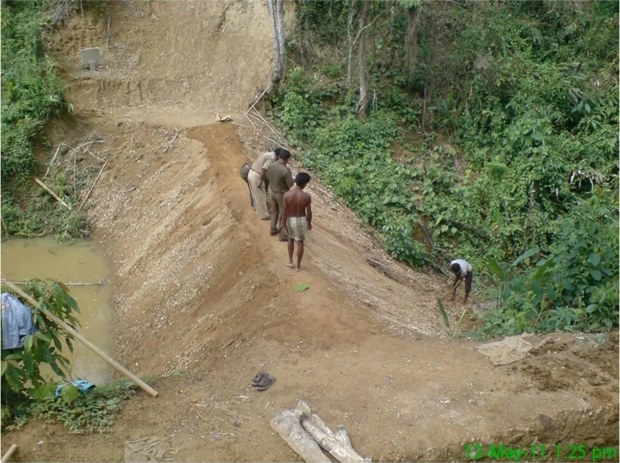
Figure 5 Check dam under construction
