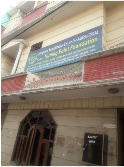
Road view of the center
